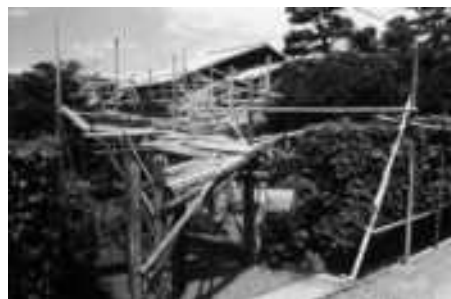
Construction "Hien So" , 1988 Work in situ, Hien So. Scrapped wood. © Photo Tetsuzo Kosaka
